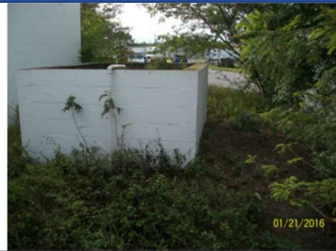
Photograph 14: Sand filter outside Southwest corner of building at
