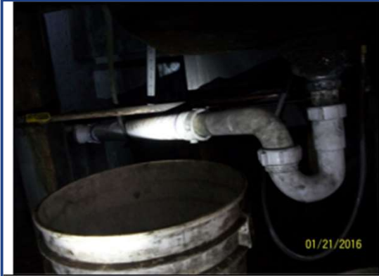
Photograph 6: Plumbing under sink leads to west wall.
