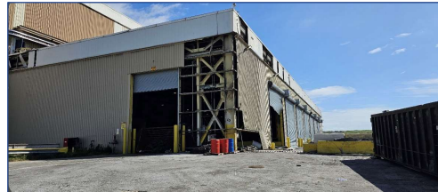
WTE Facility post-Milton
